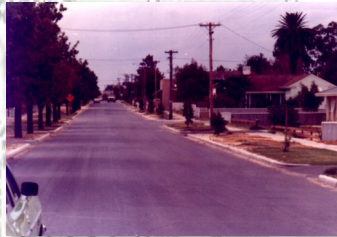
West Road after reconstruction, looking north from Bridson Street. C.1980
