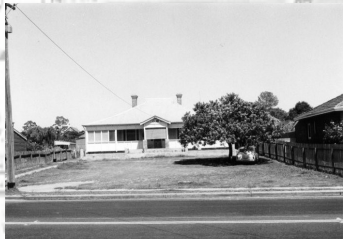
Alfred Smith's house, prior to demolition for the Bassendean Square Shopping Centre, c.1970.
