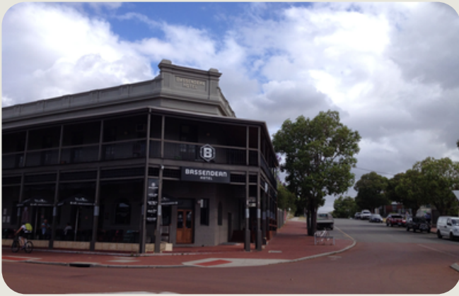
P1677 - BASSENDEAN HOTEL (DOWN OLD PERTH ROAD WALK)
