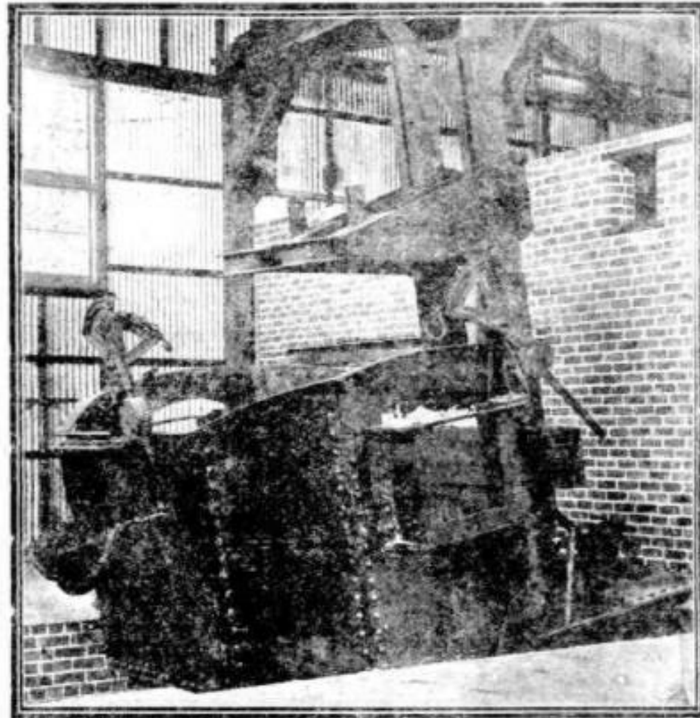
1,000-horse power electric furnace in course of erection at the Aust. Electric Steel Co.'s Works, West Guildford
